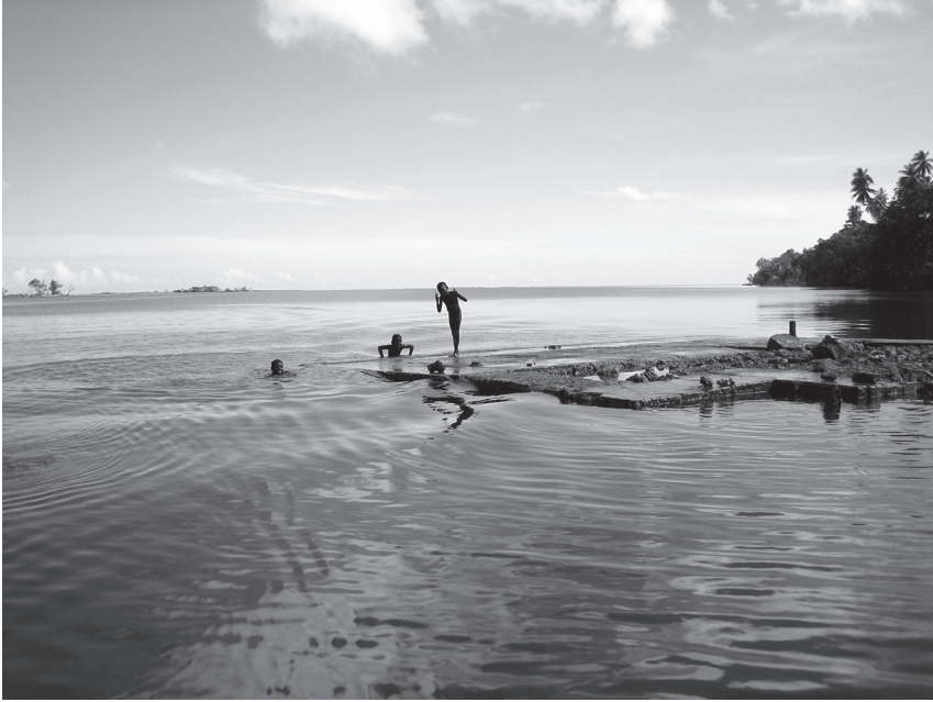
Figure 3. Children playing on Simbo's main wharf in 2011. The earthquake caused Simbo to sink more than half a meter, so the wharf became partially submerged during high tides. It was rebuilt to be above sea level by the national government several years later. (Photo by author.)
